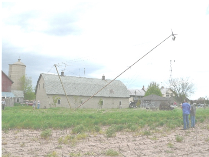
The 10 footer turbine gently rises into place, as thunderstorms off Lake Michigan loom. Each pair of observers has been assigned a specific task during the raise – everyone else is watching from outside the 'fall zone'.
