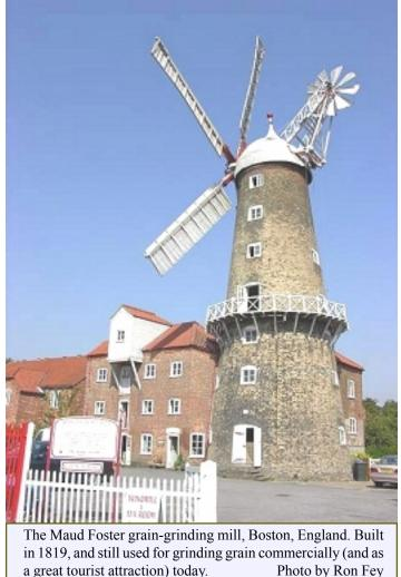
The Dutch made major improvements circa 1390 AD by incorporating lift into the blade design. The machine was pointed into the wind manually by the operator.
