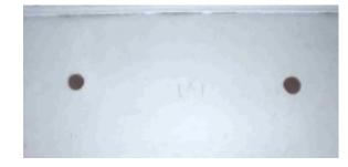
After you have a hole, you can use a probe, such as a section of metal coat hanger wire, to verify the spacing inside of the wall. Upper holes are best drilled at about a foot from the ceiling. Lower holes can be two or three feet above the floor. There will also be practical considerations that will dictate variations. Bathroom tile is one. Another may be paneling below chair rails. With kitchen cabinets, you may choose to drill from inside of them.
